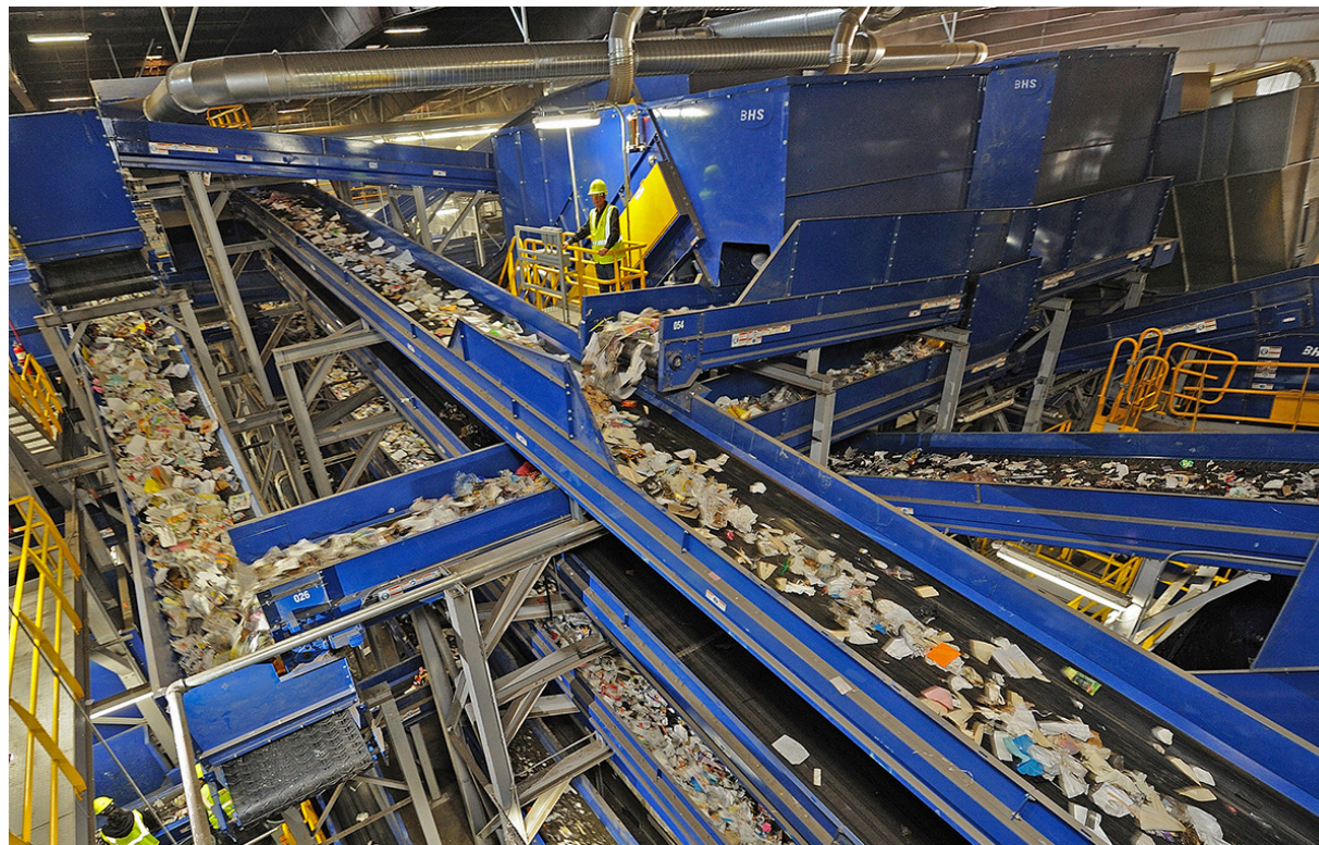
Materials Recovery Facility (MRF)
